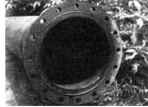
Flanged Joint, showing Gasket in groove
