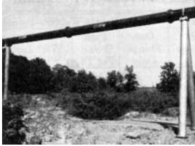
Installation of Clow Long Span Pipe
